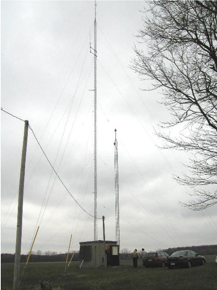
The left picture shows the repeater 110 foot tower to the left of a 40 foot tower with a wind driven electric generator used for AC power to supplement Edison. The repeater tower already has the 1200 MHz loop yagi installed just below the side mounted existing antenna for the Springfield repeater.
