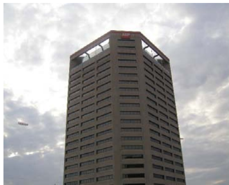
Above is the 33 story AEP building which we mounted a single remote controlled camera on the roof. A "WU80 cantenna" is pointed down through the skylight area and toward the Police building across the street.
