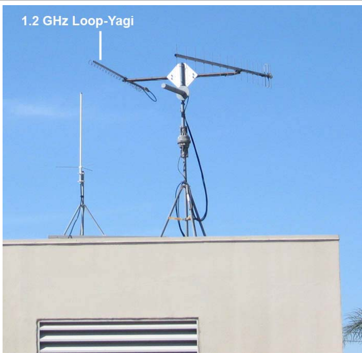
Figure 3 – 1.2 GHz Loop-Yagi on roof of OPD
