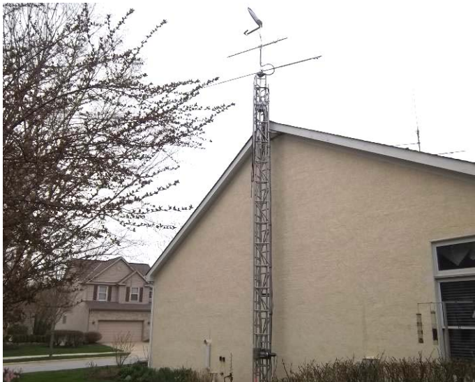
This is the south house side view showing the tower fully retracted. The antennas are top to bottom: 10GHz dish and feed, 1280MHz loop yagi, 439MHz M 2 21 element yagi.
