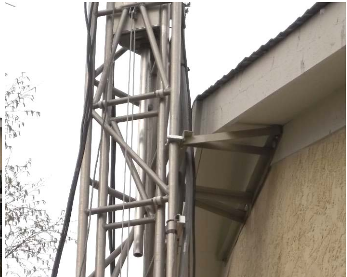
This shows the house bracket to tower connection points. The rotor is partially viewable at center top.
