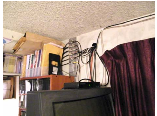
Figure IV.1 Before: I located the PolyPhaser panel above a bookcase, next to the wall pass-through. The Ham Shack is down and off to the left. The 80-meter and seismometer feed lines are long and unwieldy.
